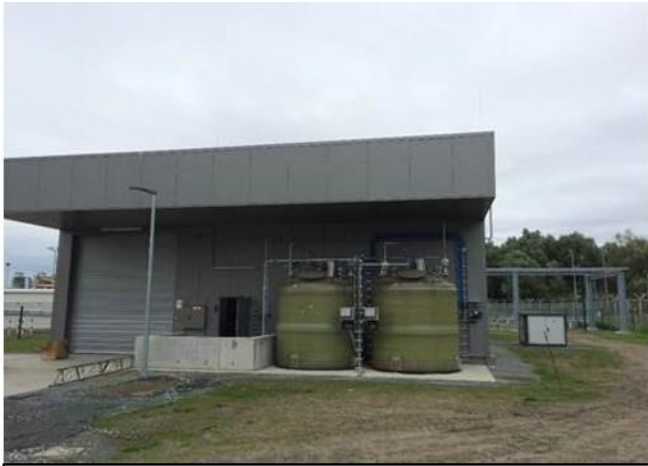
Site works completed
